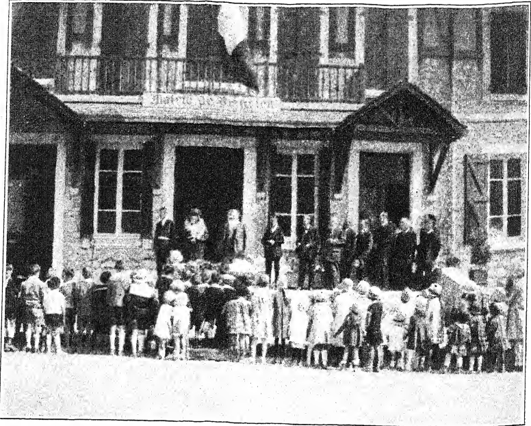
SCENE AT OPENING EXERCISES AFTER SCHOOLHOUSE WAS REBUILT AT PEYRIEU
